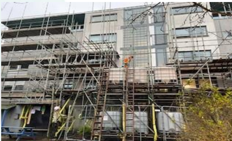
Phase 2 scaffolding ongoing
